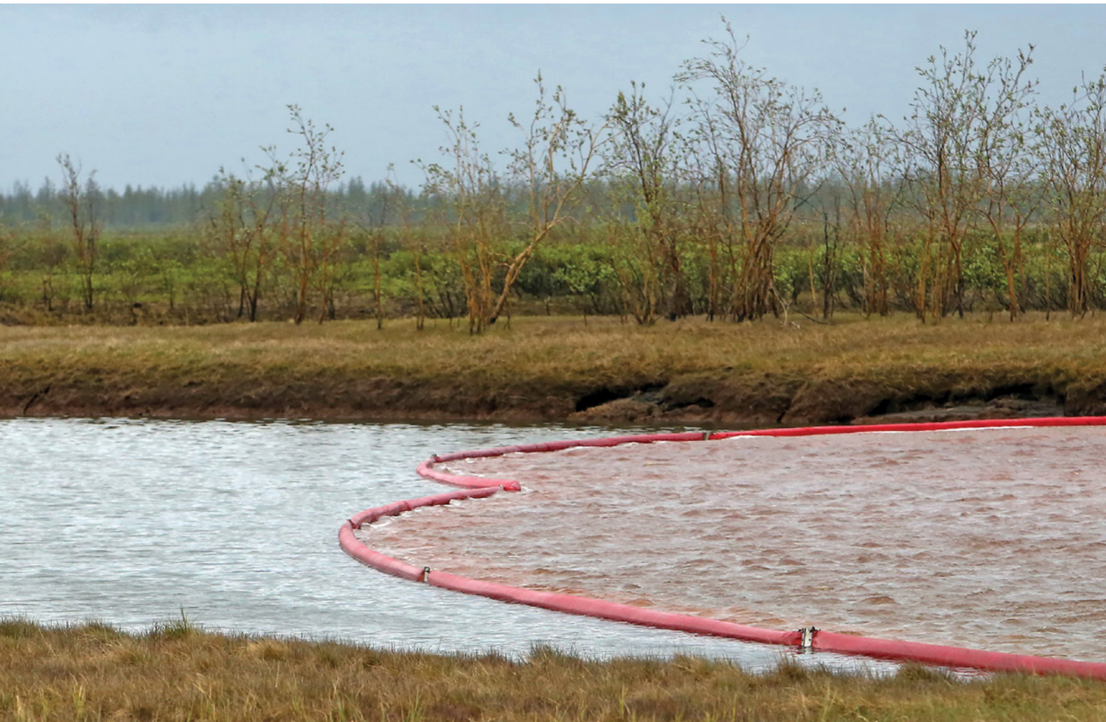
A floating dam limits the spread of oil from a massive spill in the Ambarbaya River outside Norilsk, Russia. AFP/GETTY IMAGES
