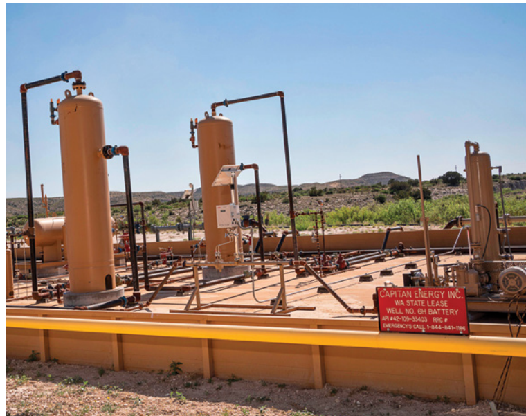
Fracking equipment stands at a Texas well in the United States. The U.S. shale gas revolution, driven by hydraulic fracturing technology, has undercut Russia's use of energy as a geopolitical weapon. AFP/GETTY IMAGES
