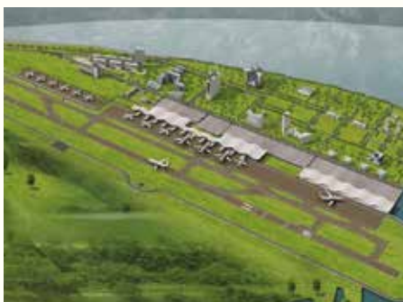
The new 10,700ft-long runway at Cox's Bazar will allow much larger aircraft to take off and land at the airport
