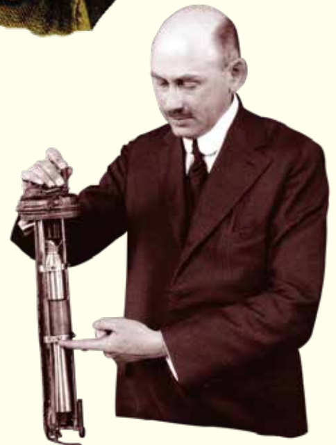
► Photo 1 October, 1924. Professor Robert H. Goddard, instructor of Physics at Clark College of Worcester, Massachusetts is shown with the first rocket he experimented with, charged with gun cotton.
